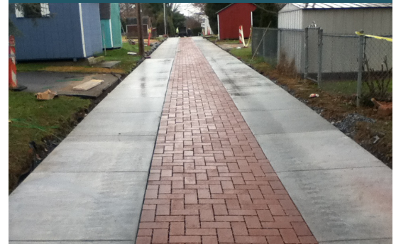
Alley 148 pervious pavers City of Lancaster, PA
