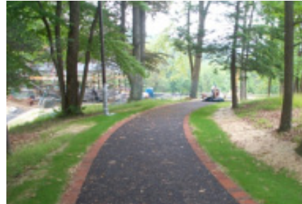
Porous asphalt path at Gray Towers National Historic Site, PA
